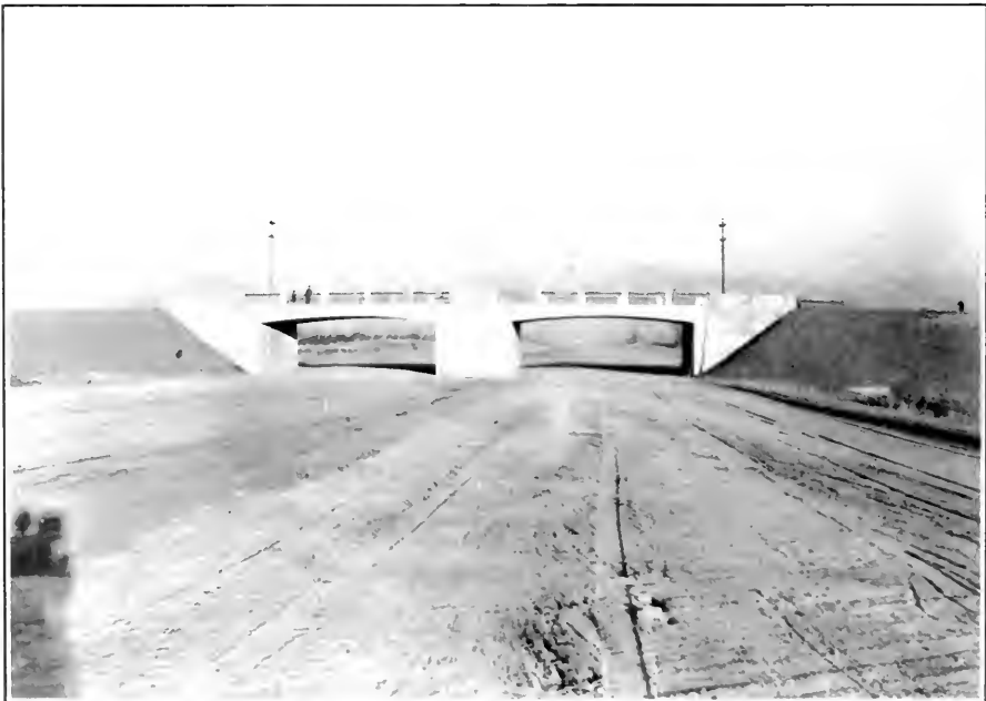
Queen Elizabeth Way Kipling Avenue Overpass, near Toronto
